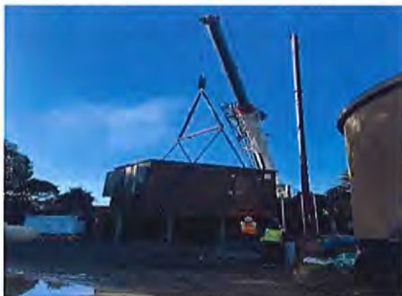
Muir Beach shelter being lifted into place.
