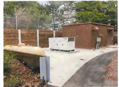
Mill Valley water tank site.
