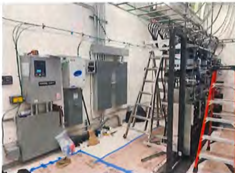
OTA Site installation in progress.
